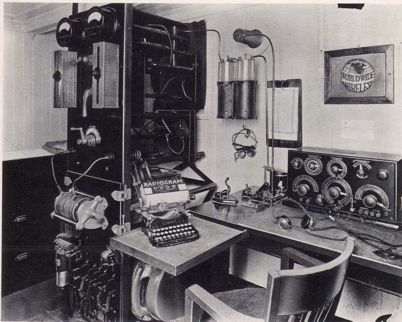
A typical 1920's shipboard spark gap transmitter (RCA P-8, 2KW) and carborundum crystal receiver (RCA-106D). Picture supplied by member Frank Geisel.
