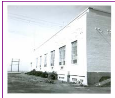
CAA Transmitter Station at Belmont, CA 1948
