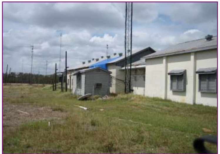
Wing of WLO TX building & Antenna Field
